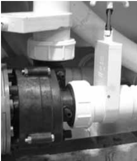
Slice Valve and Pump Union
