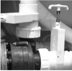
Slice Valve and Pump Union
